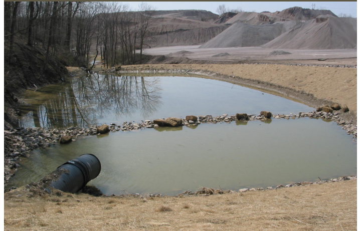
Jaymar Steel Slag Leach Bed, Photo by Brett Laverty
