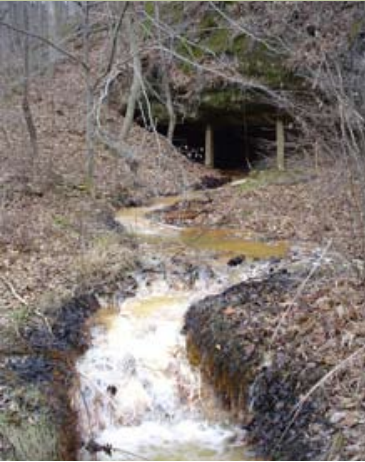
Essex Doser, Photo by Monday Creek Restoration Project
